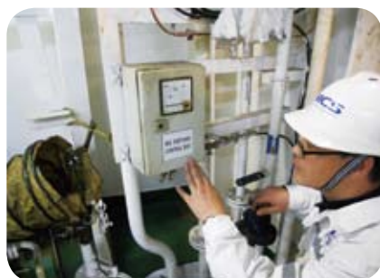
Inspection for shaft earthing
