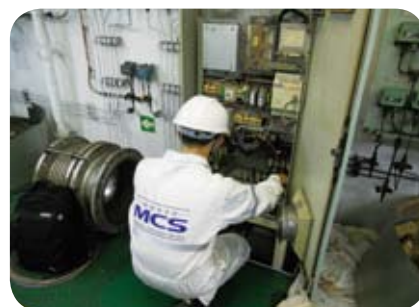
Fault finding on the ICCP power unit
